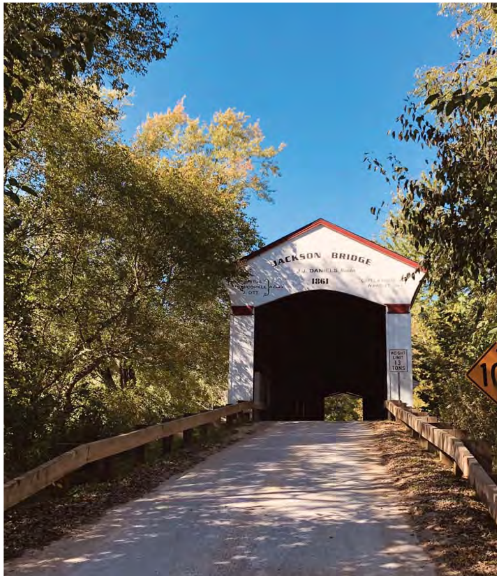
Built in 1861, Jackson Bridge is the oldest standing bridge in Parke County.
